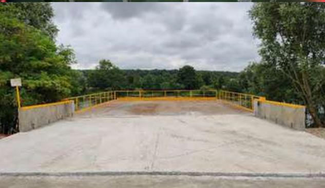
*Renovation of piles for the dolphins, creation of dolphins equipped with fenders and bollards. Demolition and removal of the platform and the outer wall in reinforced concrete. Supply and installation of a metal platform with guardrail, stop on one side, service ladder, pouring of an access slab.*
